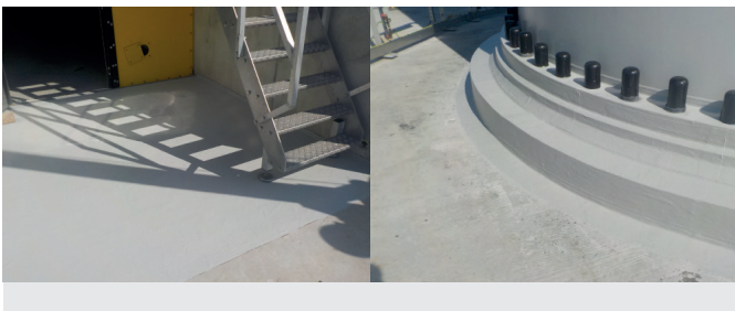
Sealing of pedestrian area and tower pedestal
