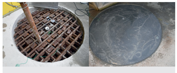
Grouting of joint between steel structure and concrete transition piece (TP) - Offshore at Nissum Bredning
