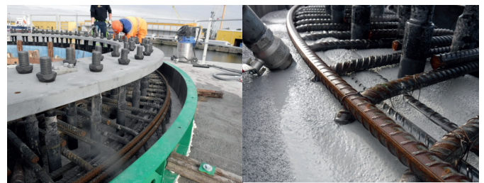
Grouting of base flange at pedestal in Poland
