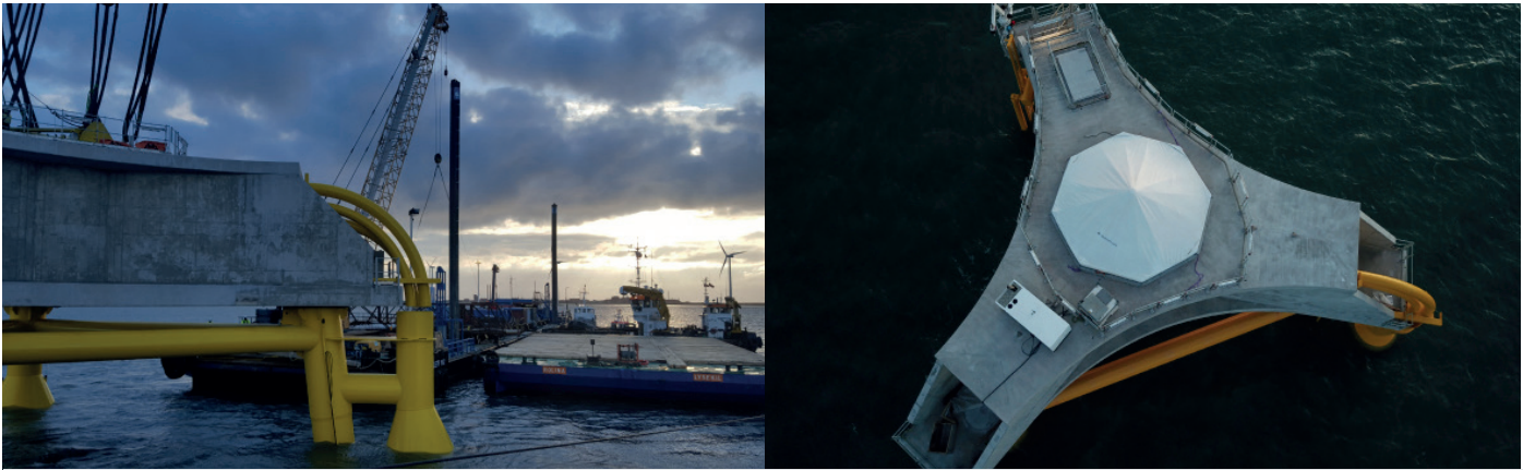
3-legged jacket with concrete transition piece
